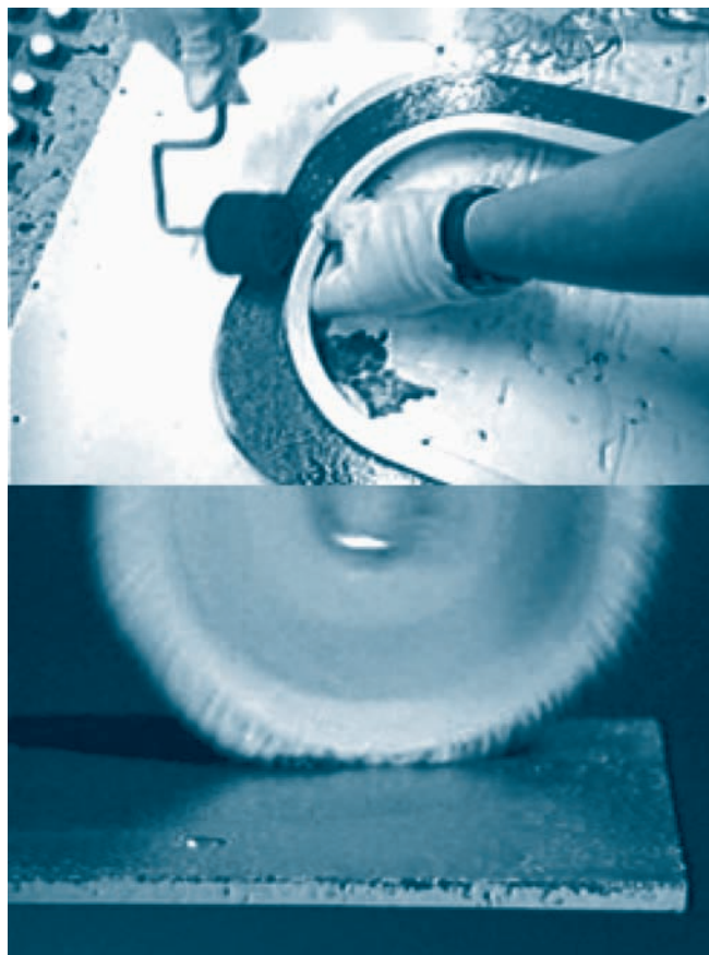
图2 装配前密封涂胶工艺 Fig.2 Seal coating process before assembly
